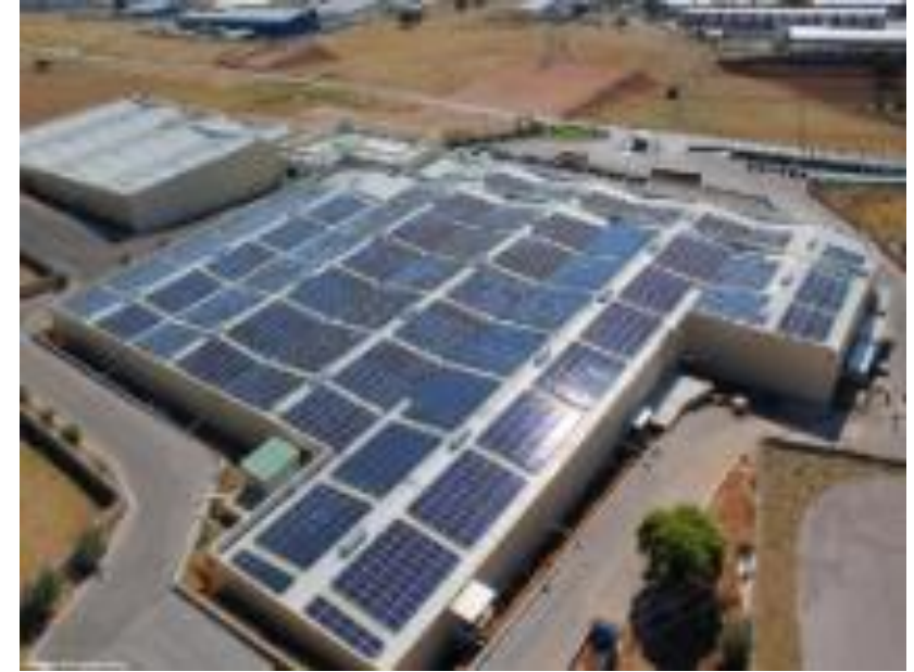
PV system of 1 MWp in Aspropyrgos, Attica
