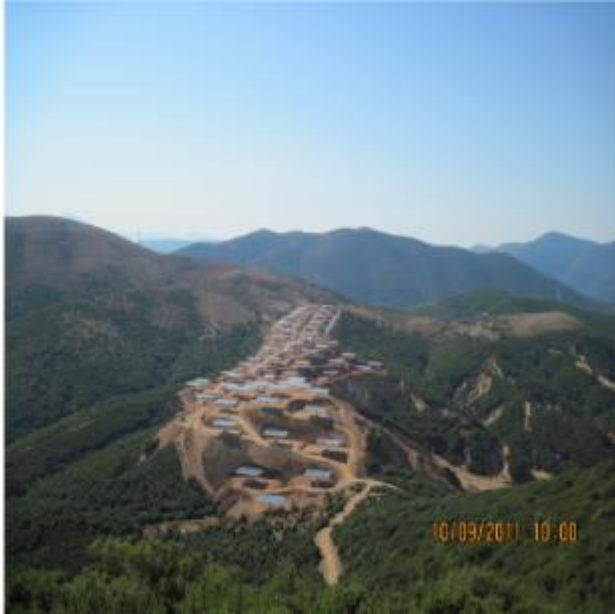
PV system of 2 MWp in Thesprotia Prefecture
